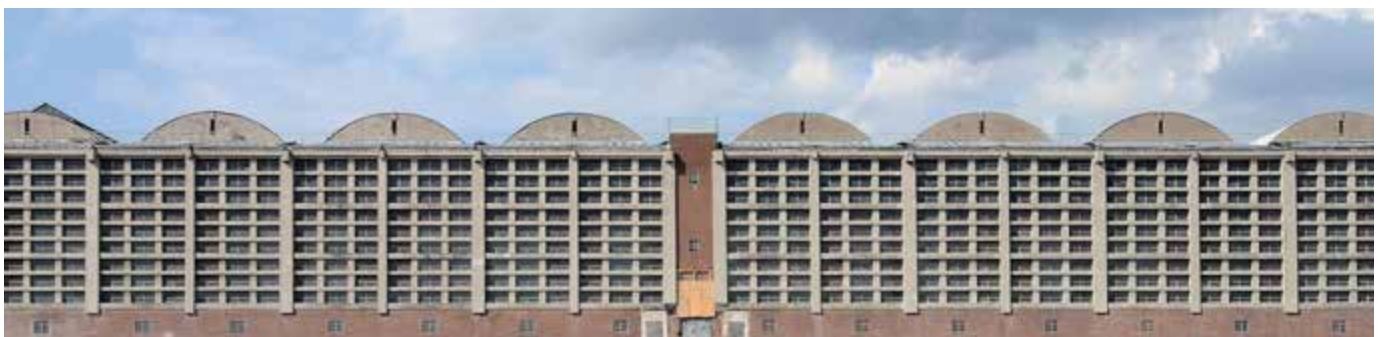
Abb. 9: Markthalle Frankfurt a.M. (Foto: Dicleli)
